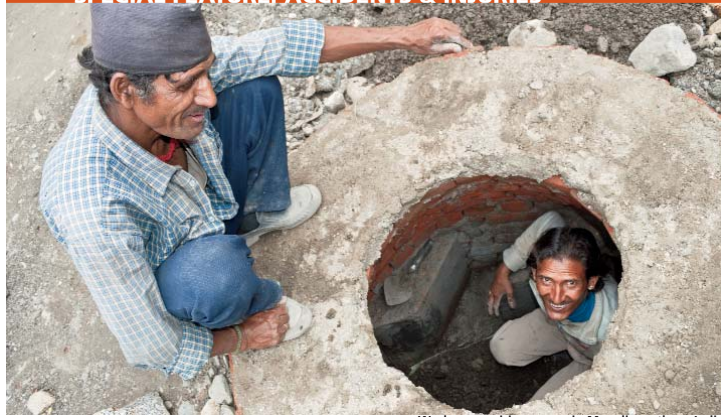
Workers repairing sewer in Manali, northern India
