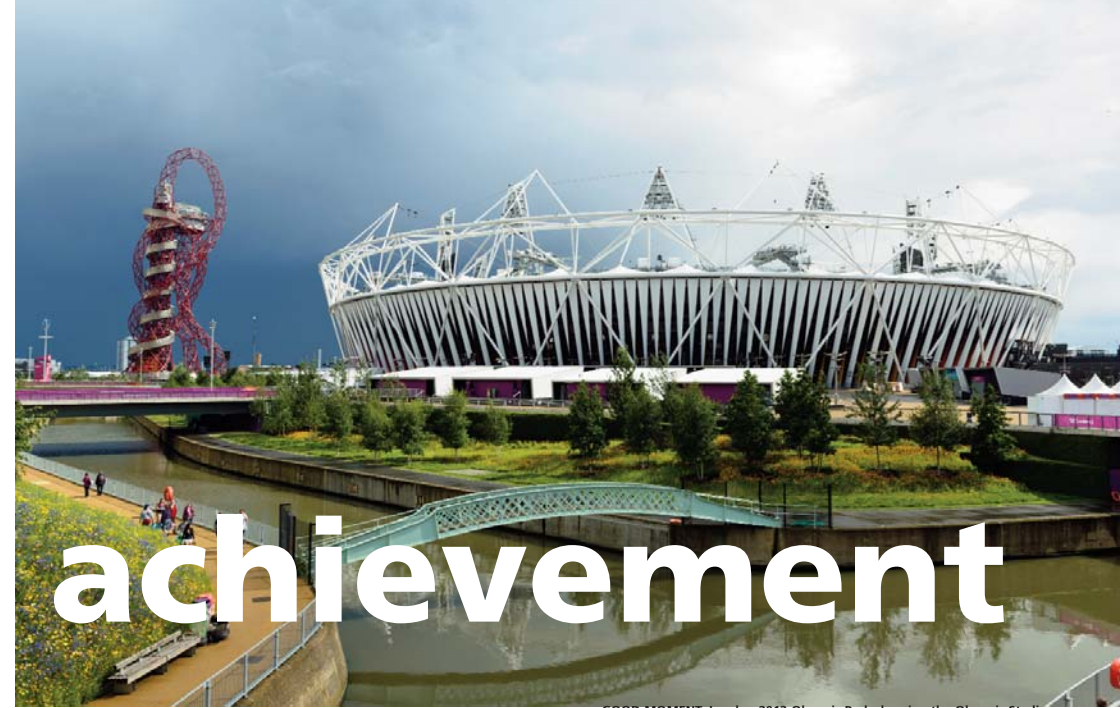
GOOD MOMENT: London 2012 Olympic Park showing the Olympic Stadium
